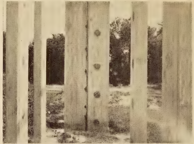
FIGURE 4.—GENERAL VIEW OF THE COLUMNS ON WHICH PRESSURE MEASUREMENTS WERE MADE
